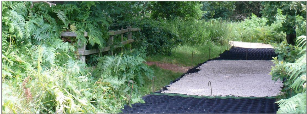
Figure 5.4: Photograph showing the installation of a cellular confinement system specifically designed for tree root protection
